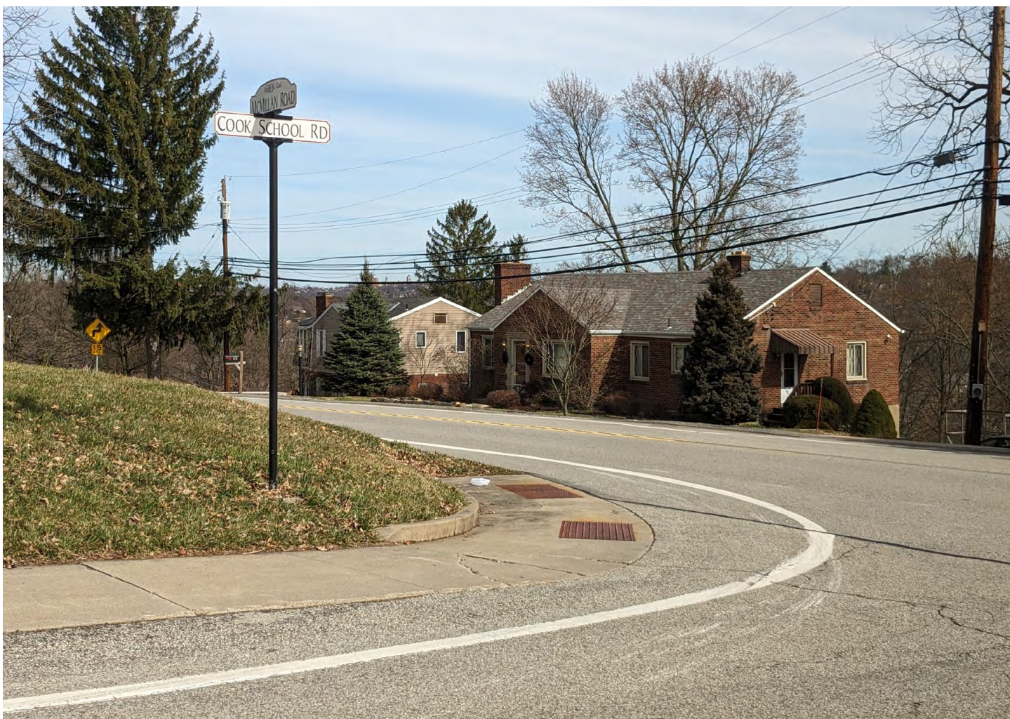
Sidewalk gaps in residential areas like at the intersection of Cook School Road and Mc-Millan Road pose as barriers to complete Township connectivity
