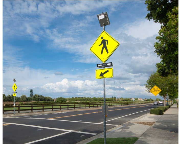
An example of a RRFB being implemented to create safer pedestrian crossings
